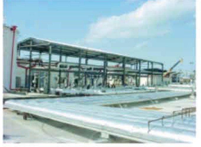
Thermal insulation works of piping
